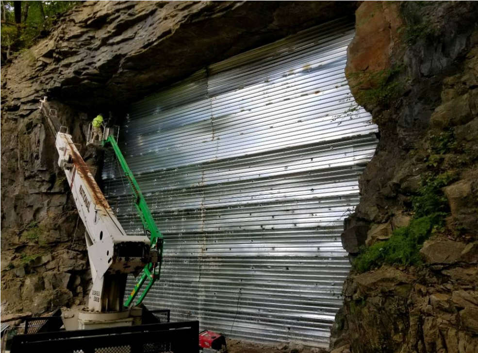
Figure 4A. Completed air dam barrier at mouth of Dunbar 1.
