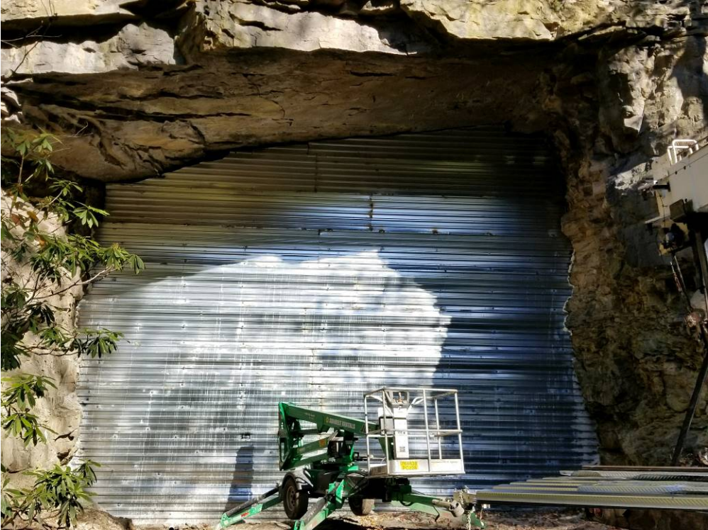
Figure 4B. Completed air dam barrier at mouth of Dunbar 2.
