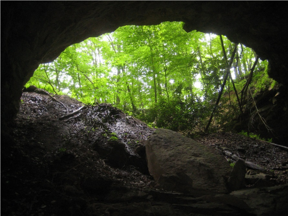
Figure 2. View looking out ceiling subsidence inside Dunbar #2.
